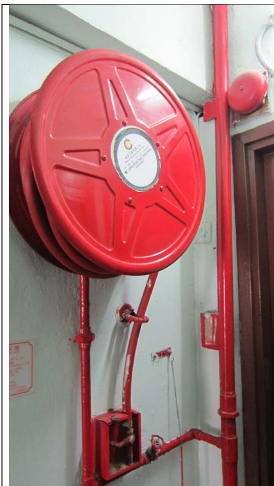
Fire services installation (hose reel)
