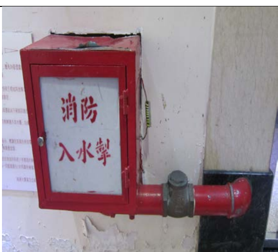
Fire services installation (fire services inlet)
