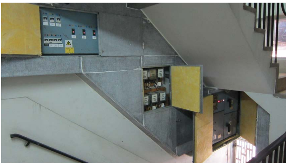
Certified distribution boxes and electric meters
